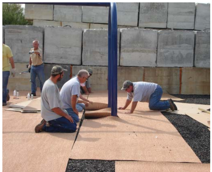
The base layer of crumb rubber has been installed. The top layer, a rubber mat system, is fit around equipment and the seams are joined. Both the equipment and surface system at this site will be installed by the park maintenance crew.
